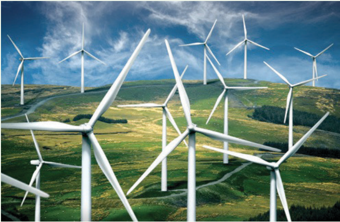
Photo Source: General Electric
